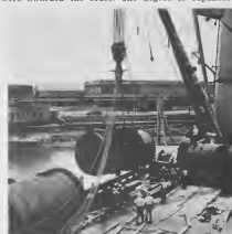
STACK SECTIONS were easily lifted off the freighter's deck and placed on a barge by the ship's crane. The Shunkoku Maru's deck crew wore safety hats.
